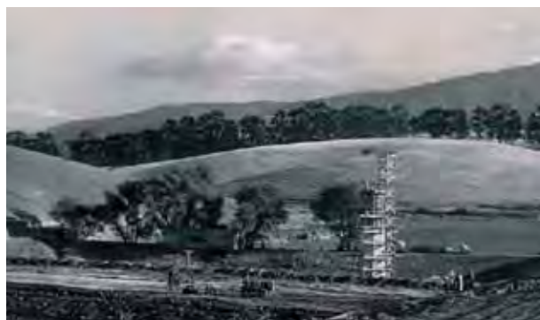
Felton Lake during construction, courtesy David Freyberg
